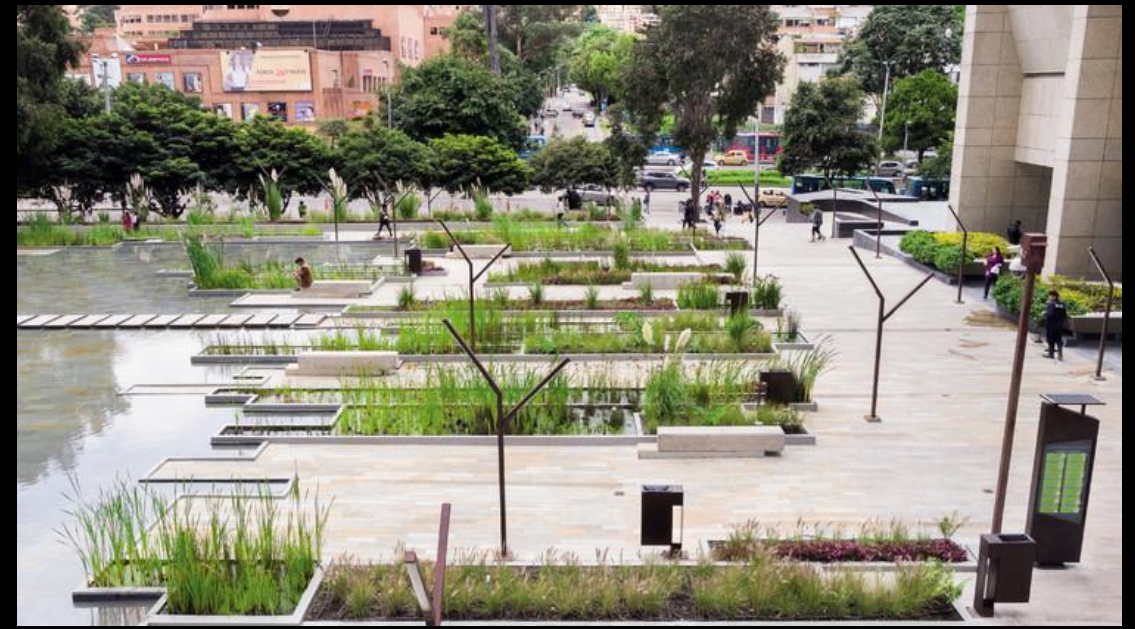
Torres Unidas Building, Bogotá
